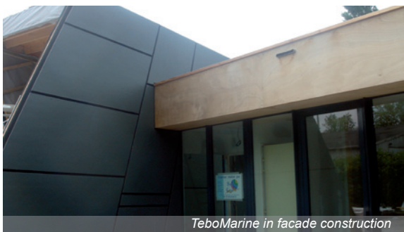
TeboMarine in facade construction
